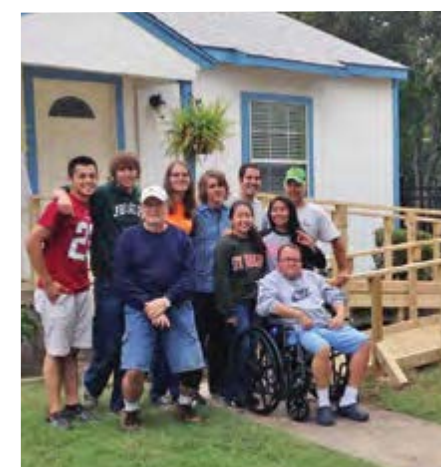
UTD Terrys build a wheelchair ramp.
