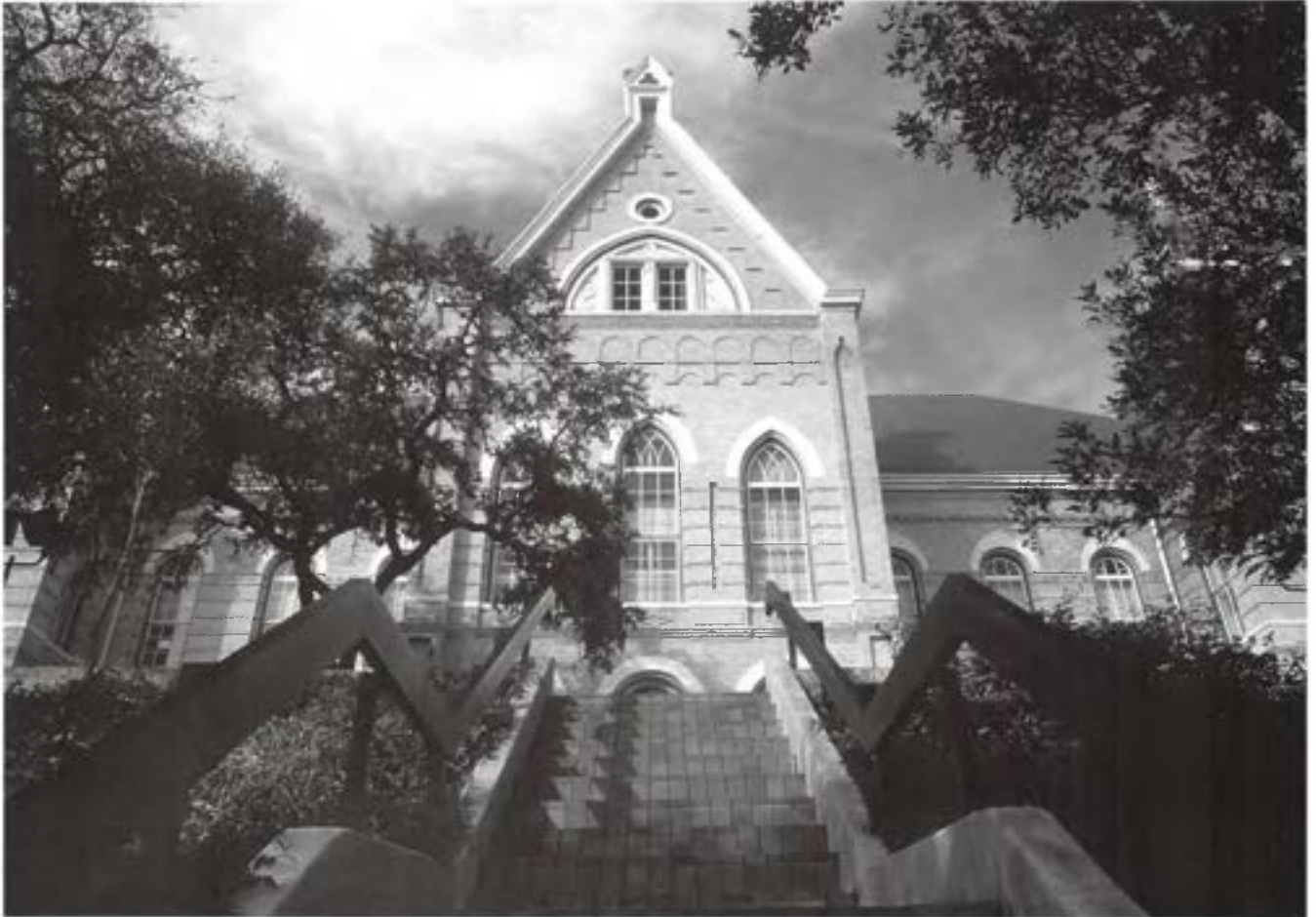
Located at the heart of campus, "Old Main" has long been the symbol of Texas State University-San Marcos.
