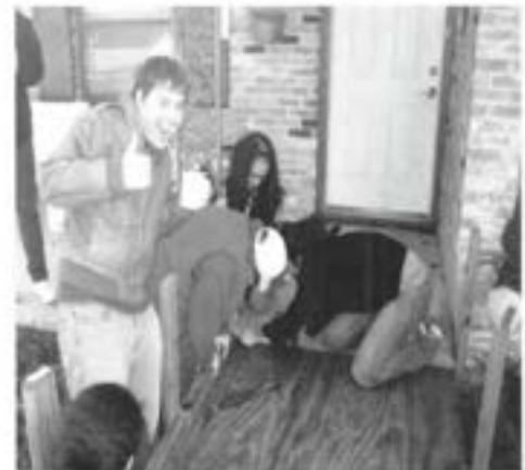
UT-Dallas Scholars construct handicap-access ramps.
