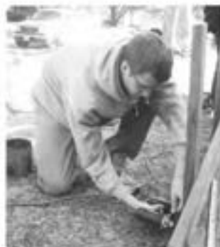
UT-Dallas Scholar Carson Curry at the Dallas Ramps project.
