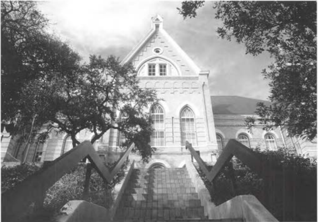
Located at the heart of campus, "Old Main" has long been the symbol of Texas State University-San Marcos.
